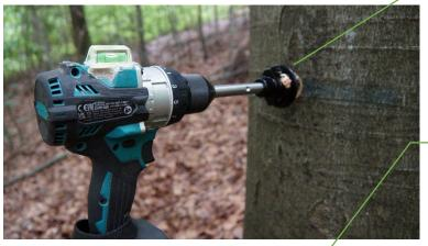
Install the first platform bolt in accordance with the installation instructions for platform bolts.
