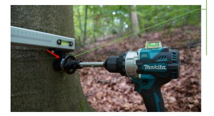
Drill the position of platform bolts three and four.
