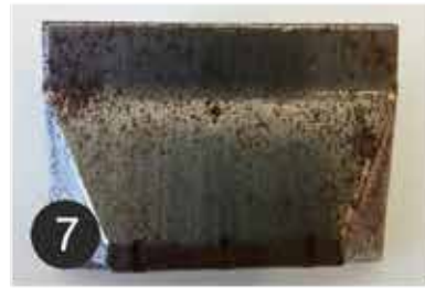
7 Corrosion check on MCD components.
