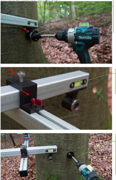
Drill the position of BABO BOLT three and four. ATTENTION the countersink must not touch the guide sleeve!
